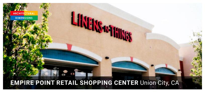
**The 84,000 S.F. Empire Point Retail Shopping Center** was designed to include two retail buildings (72,000 S.F. and 12,000 S.F.) and a pad building for Applebee's Restaurant. The buildings are masonry construction with wood frame structure.
