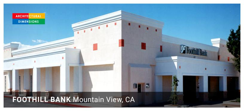
The 6,000 S.F. bank redesign was part of a 45,000 S.F. major exterior remodel of an old shopping center to capture new retail tenants. A new canopy utilizes the old structure with additional steel frames buttressing the building to mitigate structural deficiencies. Variety of stucco colors, cornice moulding and inset color tiles were added to create a new "conservative Mission" style.
