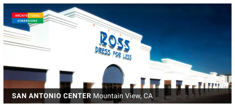
**The San Antonio Center project** included a 45,000 S.F. major exterior remodel to an old shopping center to capture new retail tenants. A new canopy utilizes the old structure with additional steel frames buttressing the building to mitigate structural deficiencies. The window systems were changed to painted aluminum, awnings, and inset color tiles were added to create a new "Conservative Mission" style.
